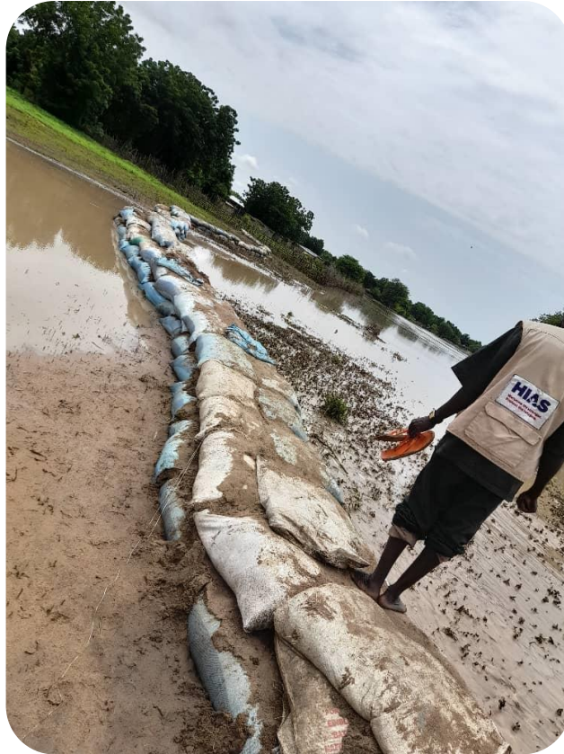
Flooding in Koukou, Chad. 2022
